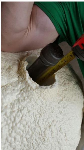
Closed Cell Spray Foam Insulation Applied
