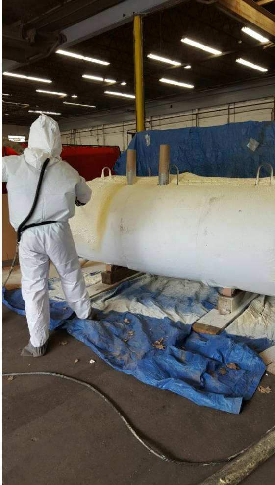
Closed Cell Spray Foam Insulation Applied
