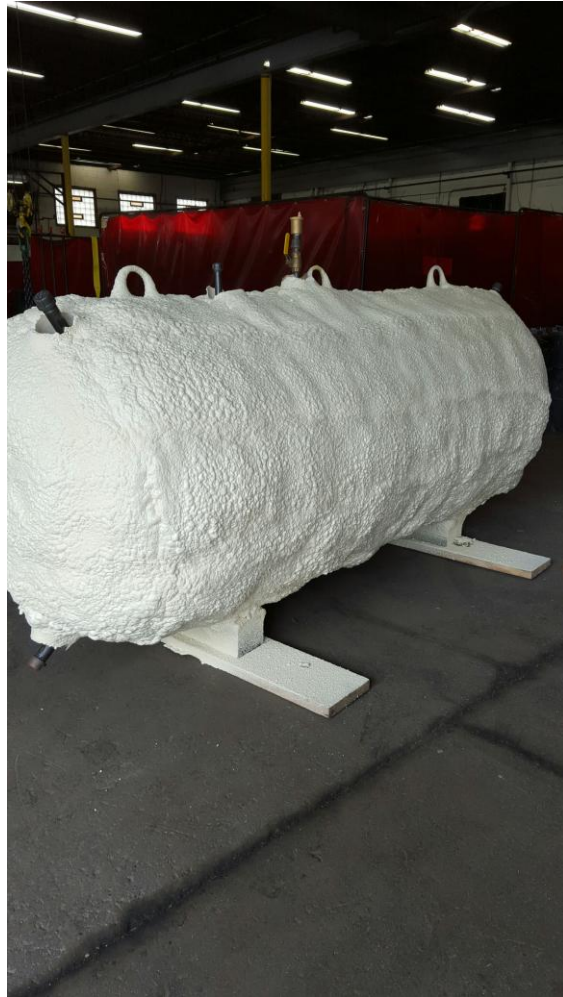
Intumescent Fire Barrier Coating Applied
