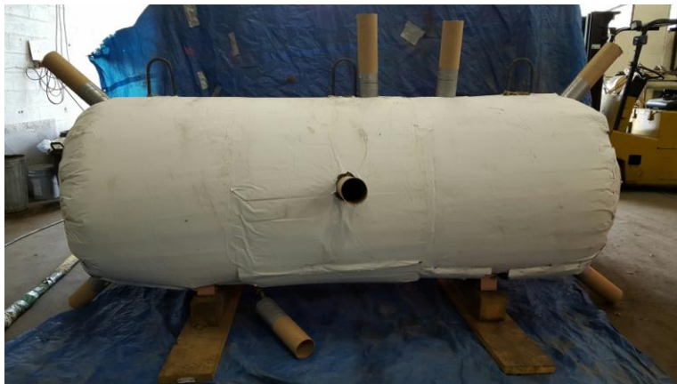
Mineral Wool Blanket Applied and Forms for Couplings Placed
